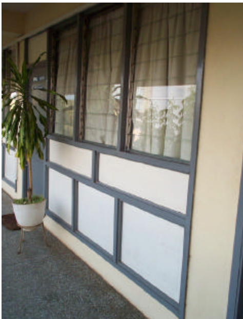
The lower louvred windows were replaced with solid flush wooden panels
