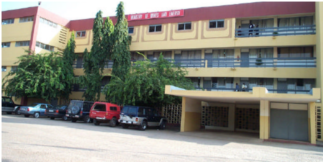
The three storey Ministry of Mines & Energy Building in Accra
