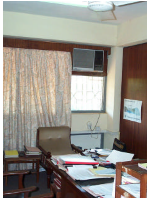
Air Conditioners were moved from the floor level to a height of 1.5-2meters.
